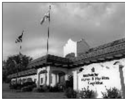
New facility of the Institute for the Interdisciplinary Study of Human & Machine Cognition in Pensacola, Florida.
